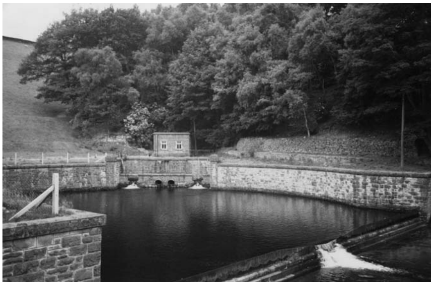
Figure 10.31 View of 120° V notch in foreground and two 90° V notches in background.
