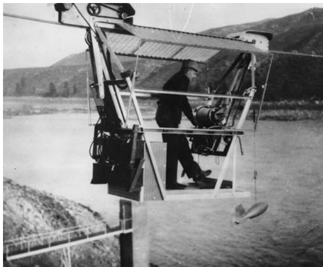
Figure 2.22 (a) Manually operated cable car with single-drum winch, cup-type Price current meter and Columbus sounding weight.
