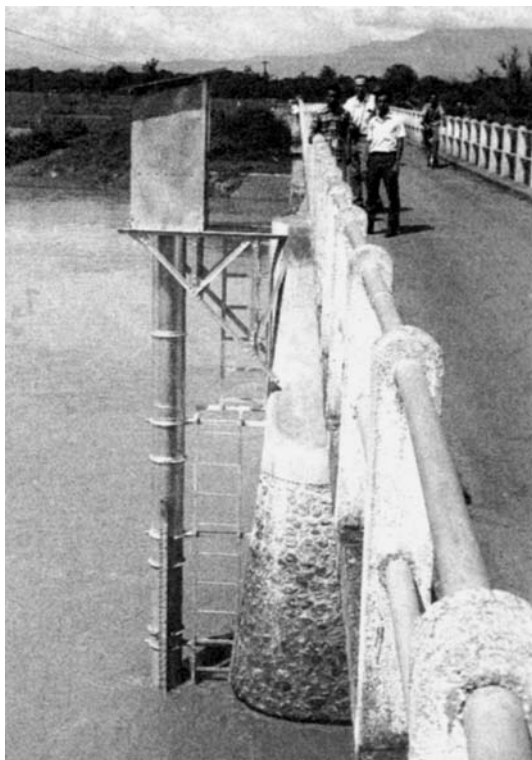
Figure 3.29 Streamflow station (Indonesia) with hung stilling well of steel pipe from bridge with 'look-in' instrument shelter and access ladders to vertical staff gauge.
