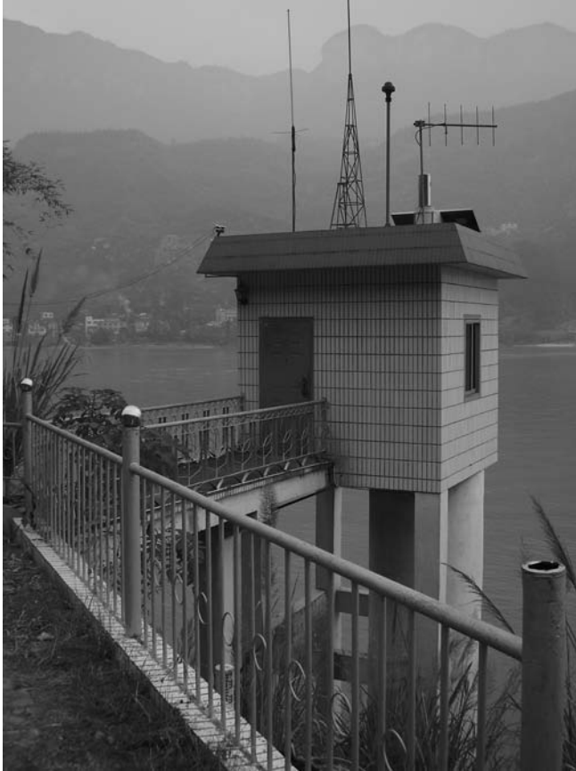
Figure 3.30 Streamflow station Yangtze River at Hueng Ling Miao, China showing instrument house and satellite and radio antennas.
