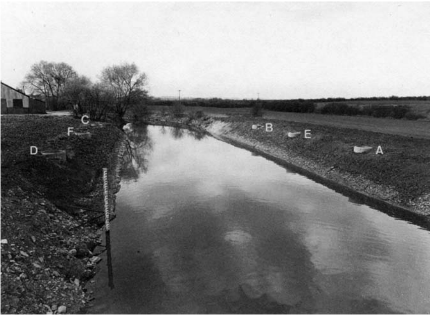
Figure 2.33 Electromagnetic gauging station: coil installed beneath river; bed insulated with insulation membrane covered with gravel; manholes A, B, C and D are installed at corners of coil and used for access to ducts; manholes E and F are at extremities of duct carrying electrode and coil cables to instrument house (not shown).
