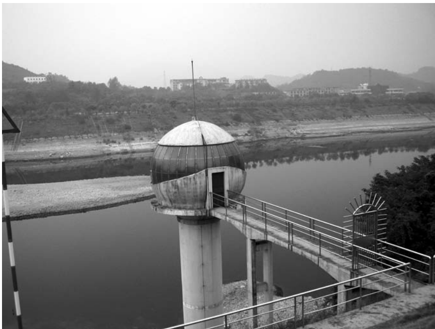
Figure 3.31 Streamflow station Qing River at Gao Ba Zhon, China showing instrument house, satellite and radio communication antennas.
