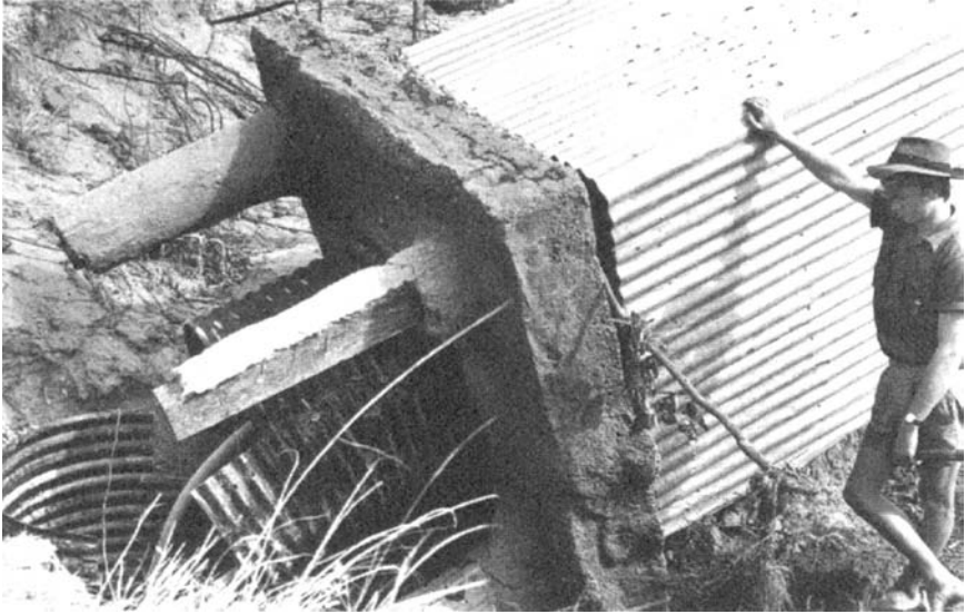
Figure 3.23 Stilling well and instrument house overturned by flood (Queensland, Australia).
