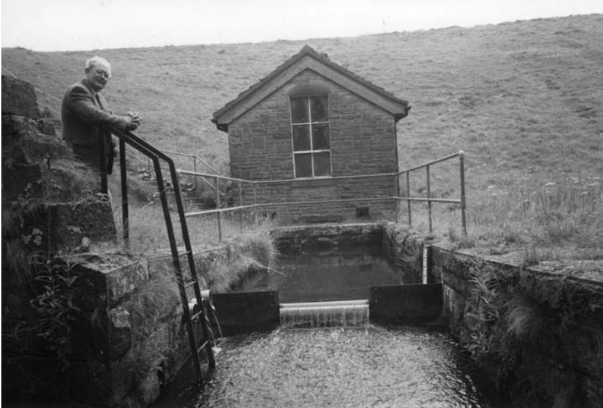
Figure 10.9(a) Rectangular thin plate notch (contracted) weir.
