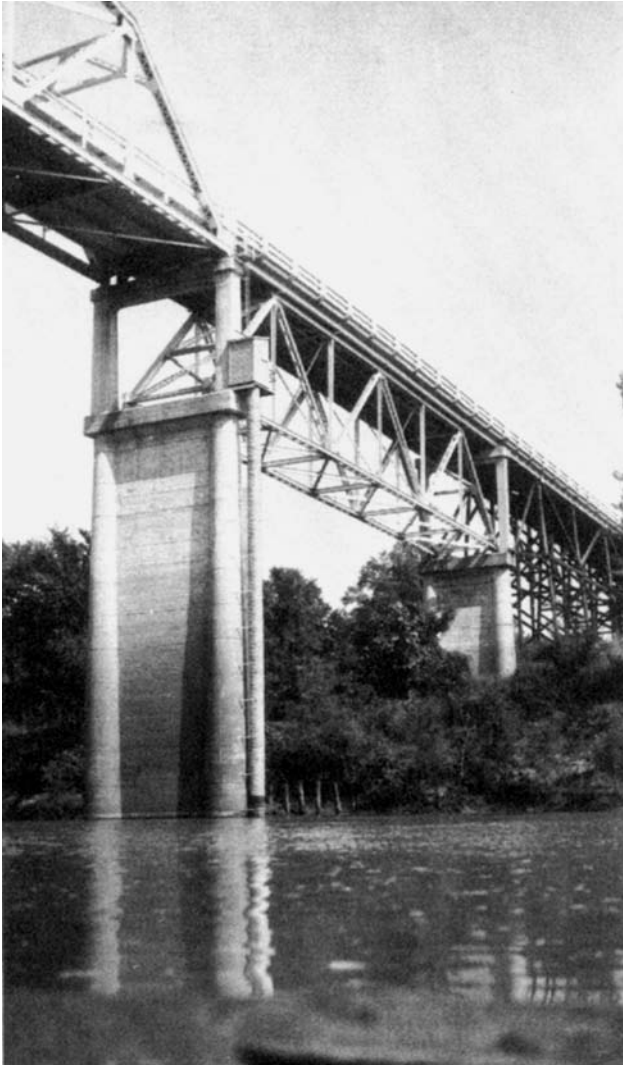
Figure 3.28 Streamflow station (USA) with hung stilling well of corrugated steel pipe fixed to bridge pier with hoop brackets.
