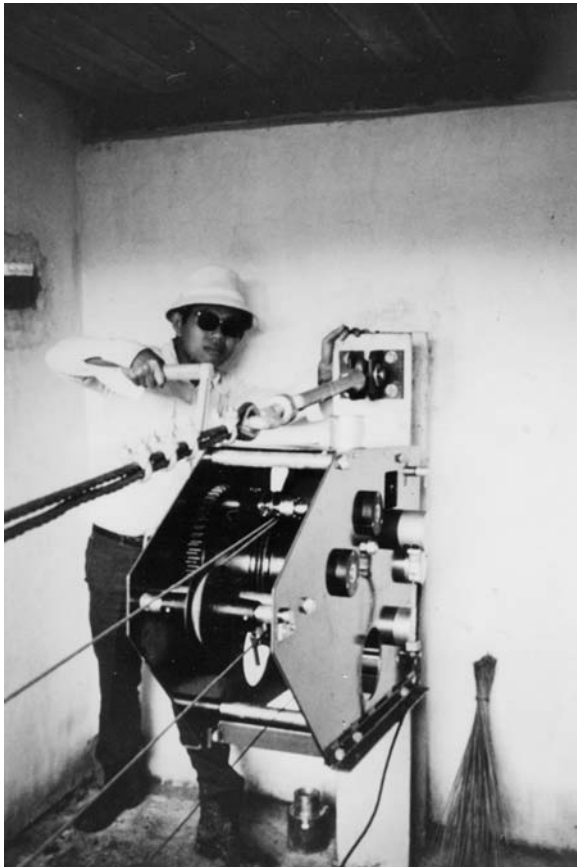
Figure 2.18 (a) Double-drum winch.
