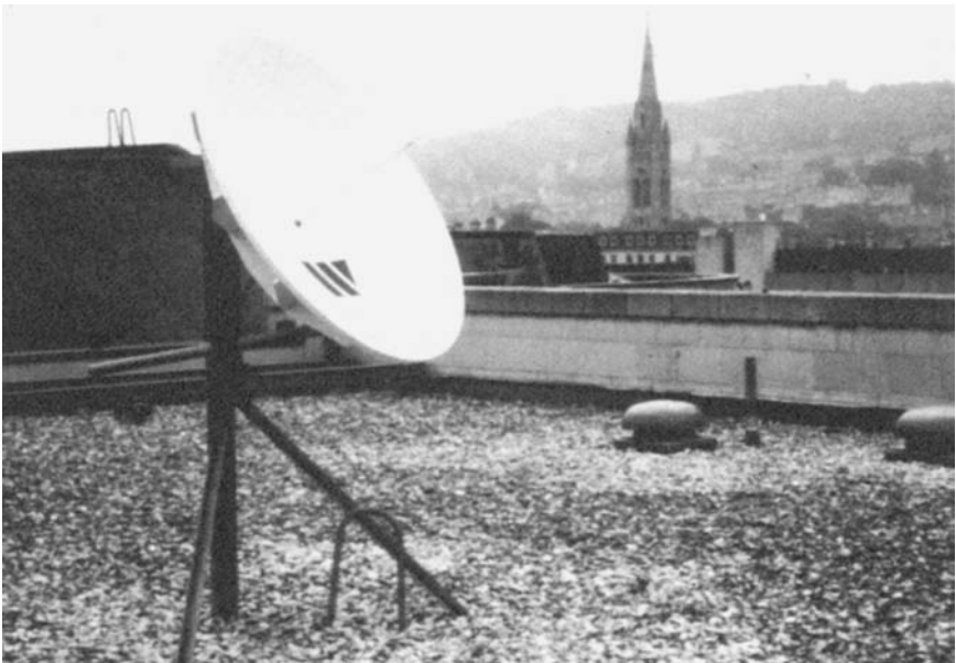
Figure 3.38 Satellite receiving dish antenna (1.5 m diameter) for METEOSAT. The antenna receives streamflow data from the satellite within 4 min. of transmission and is on-line to a central computer.
