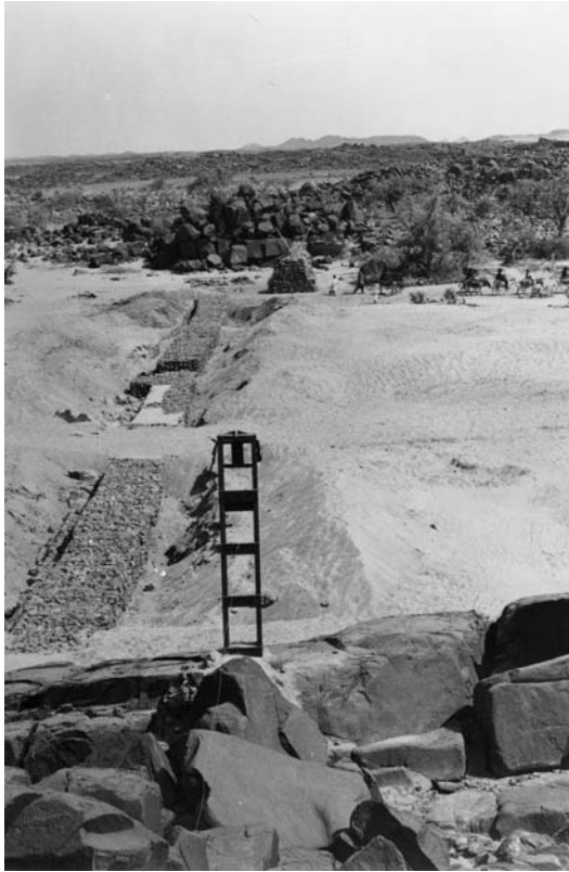
Figure 5.20 Installation of bed control using gabions in arid-zone streams.
