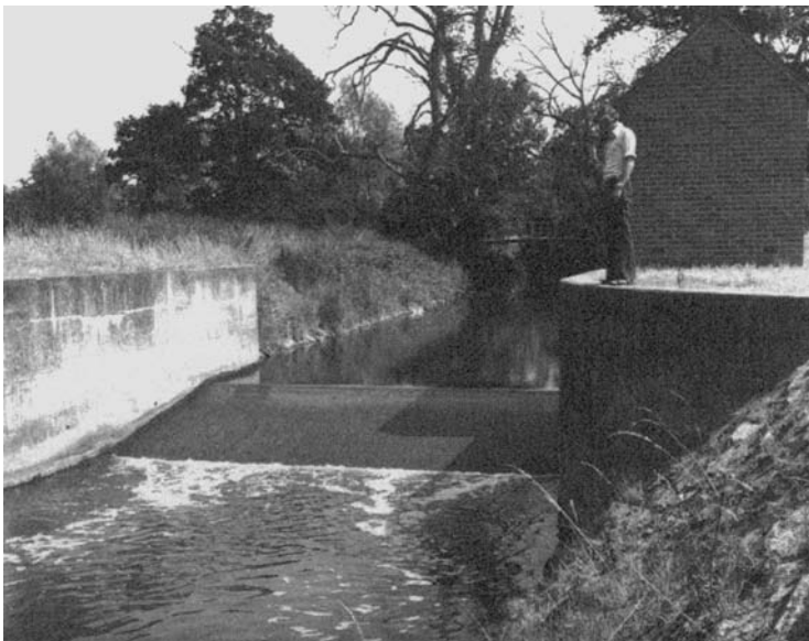
Figure 10.28 Triangular profile (Crump) weir having a single crest.
