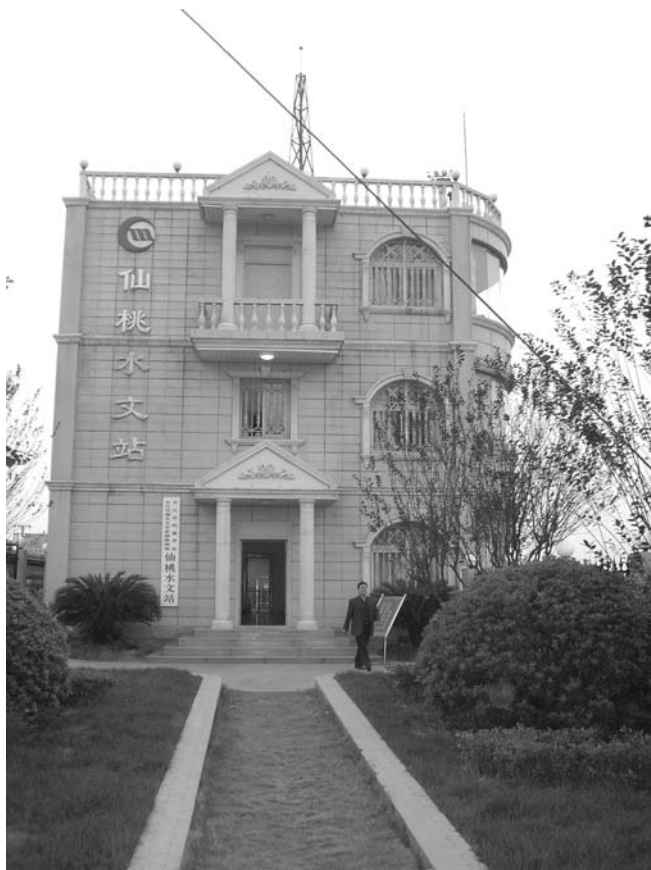
Figure 3.27 Streamflow station Han River Xian Tao, Wuhan, China, instrument house and hydrometric conference centre with satellite and radio communication.
