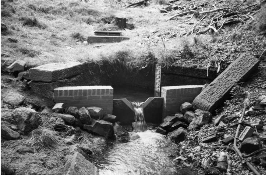
Figure 10.10 V-notch thin plate weir.
