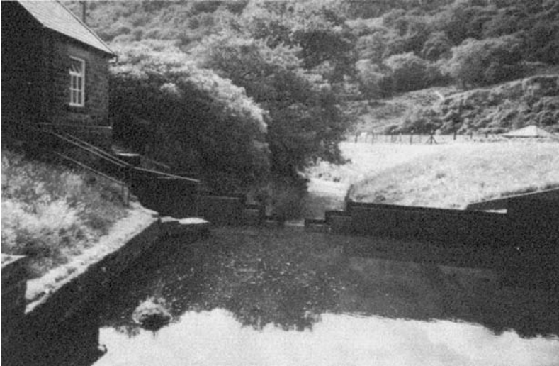
Figure 10.33 Compound thin plate weir having five crests.
