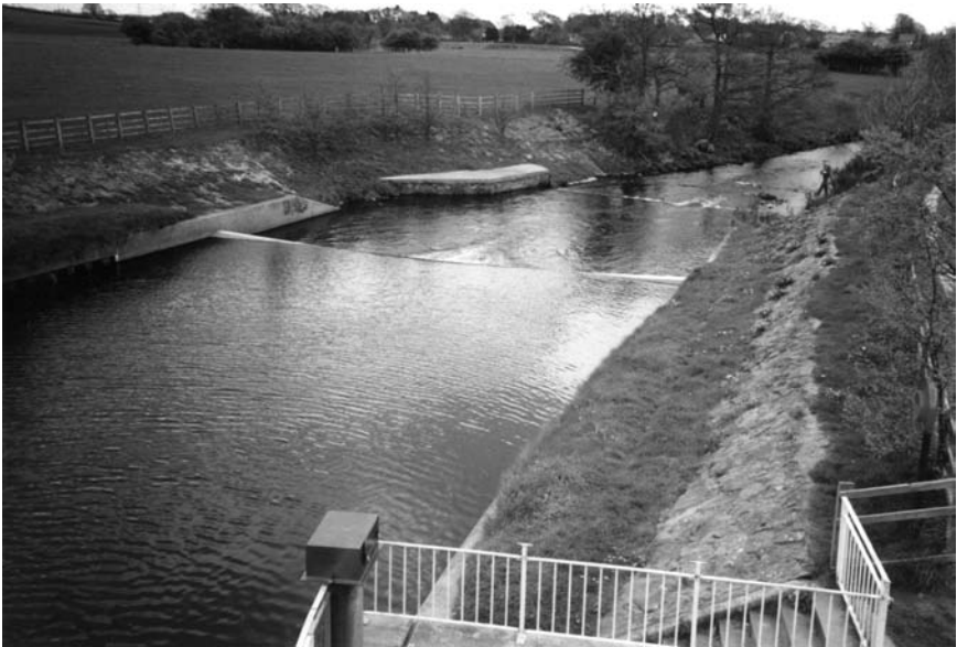
Figure 10.30 Flat V weir.
