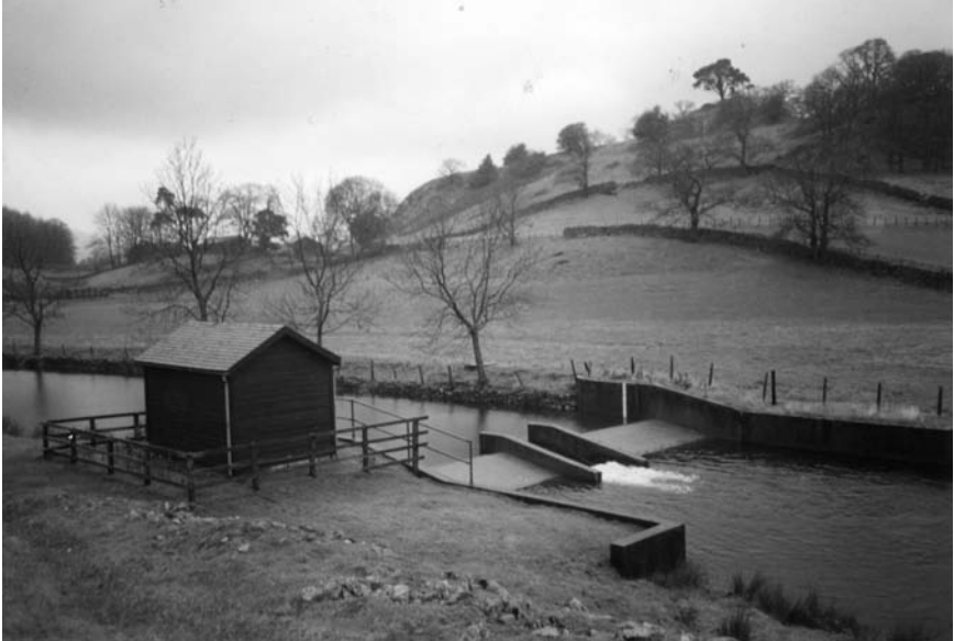
Figure 10.29 Compound triangular profile (Crump) weir having a low flow central crest and two flanking crests.
