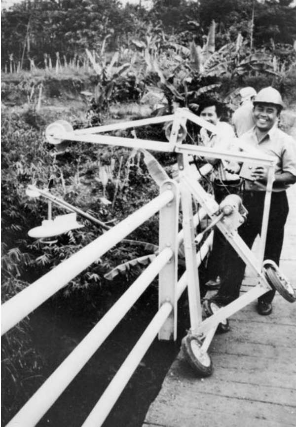
Figure 2.23 Current meter measurement from bridge using bridge crane, Java.
