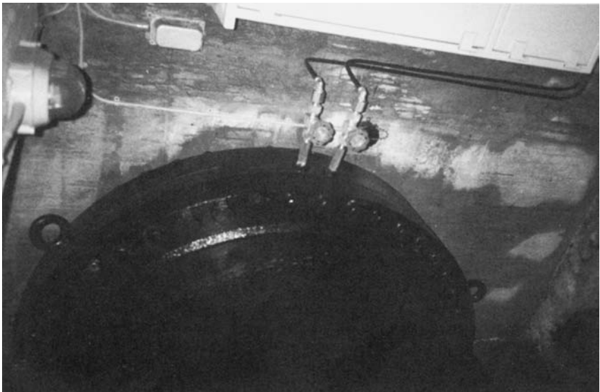
Figure 15.1 Orifice plate meter, (a) diagrammatic sketch and (b) view of meter in application.
