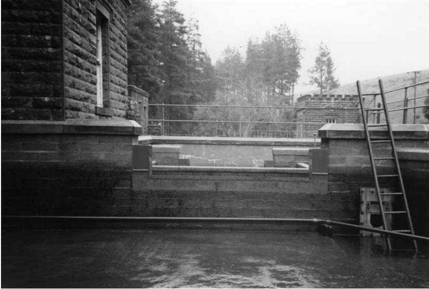
Figure 10.27 U-shaped orifice (right foreground under ladder) to measure compensation water. The head over the rectangular thin plate weir in the centre of the picture is maintained sensibly constant so that the head over the orifice is also constant maintaining a constant designed compensation flow into a side chamber for return to the river. The rectangular thin plate weir measures the flow to supply.
