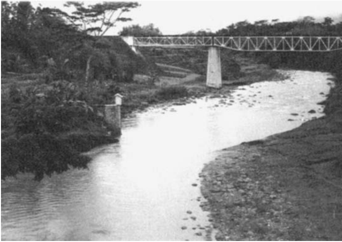
Figure 4.3 Complete section control (Indonesia) with upstream pool stable and sensitive.
