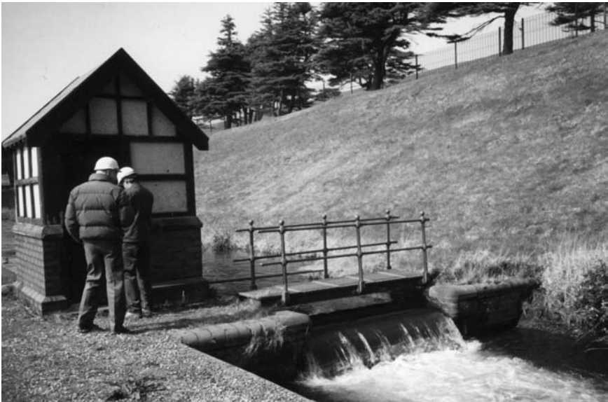
Figure 10.9(b) Rectangular thin plate full width (suppressed) weir.
